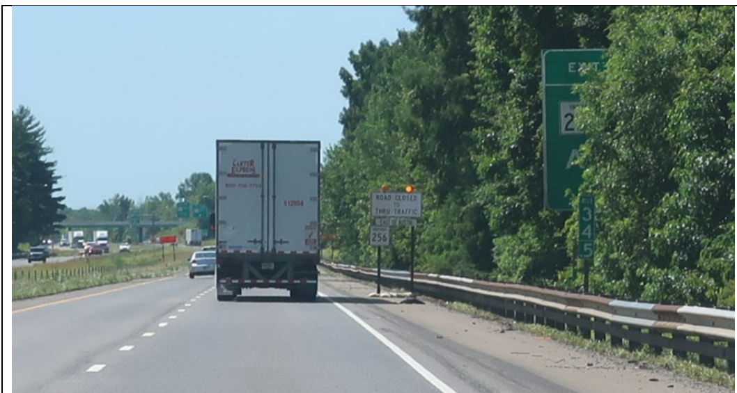
Figure 13: Example of vegetation growth reducing visibility of sign on right side of road
