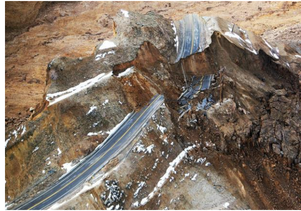
Bingham Canyon Mine Landslide, April 10, 2013
