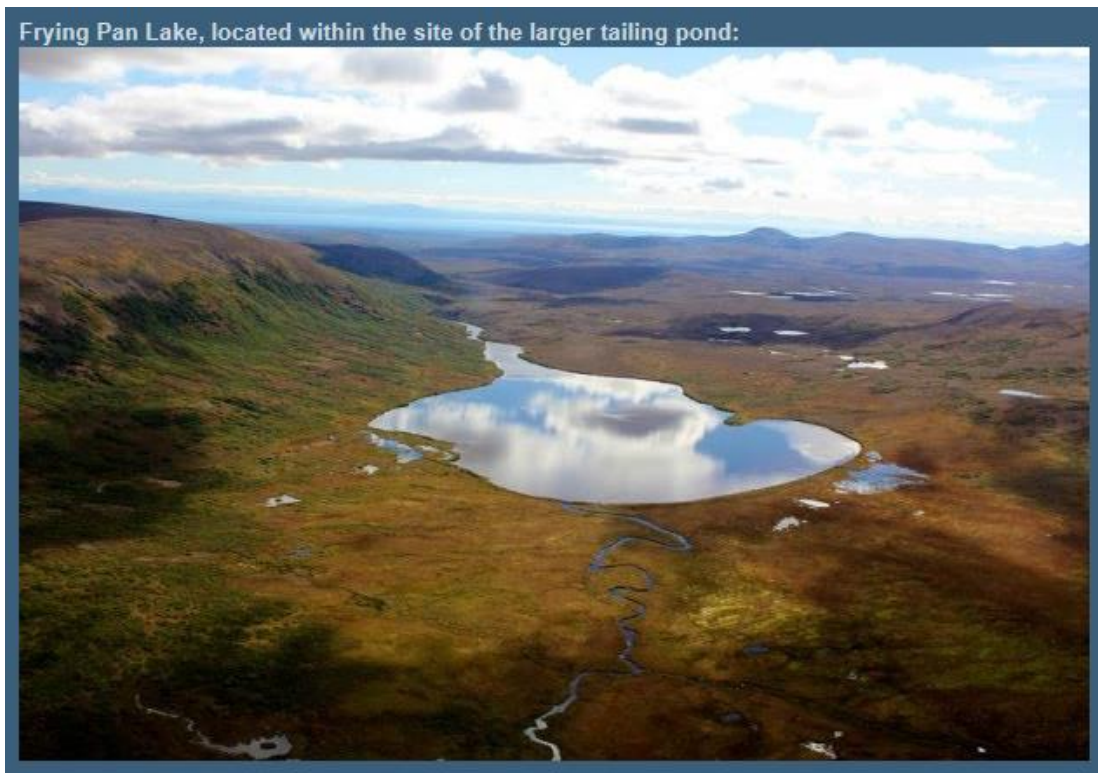
Tailings ponds used to hold waste from mining operations at the Pebble Mine site would cover an area between 10-15 square miles. The area shown above where Pebble intends to place one of its largest tailing ponds includes Frying Pan Lake which drains into the Kaktuli River and eventually Bristol Bay. [FNs]
