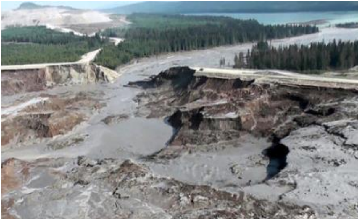
The wall of the tailings dam, that contains toxic mine waste, at the Mount Polley Mine in British Columbia ruptured on August 4, 2014, sending an estimated 8 million cubic meters of mine waste into surrounding waterways.
