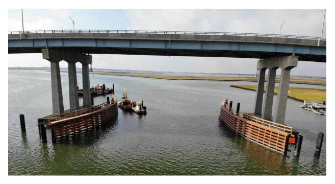
Advanced ultraviolet additives protect coastal reinforcements from sunlight and heat degradation and are coupled with composites' proven ability to withstand corrosion and structural degradation in fresh and saltwater environments. These properties allow for extended service life along with reduced maintenance costs. This type of system was used to rehabilitate the service dock at the Statue of Liberty in the wake of Superstorm Sandy
