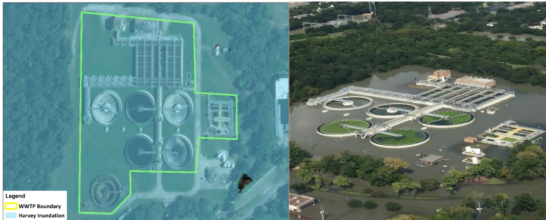
Figure 9. Illustrations of the modeled extent of flooding from geospatial modeling of wastewater treatment plants after Harvey (select facilities shown in the top figures). The bottom images compare the modeled flooding during Harvey on the left to an actual photograph taken during Harvey on the right for the Turkey Creek wastewater treatment plant
