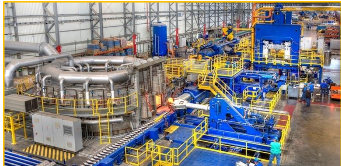
FIG. 16: Fabrication of Tokamak Cooling Water System piping is underway at Schulz Xtruded Products in Robinsville and Hernando, Mississippi. A total of 36 kilometers of nuclear grade stainless steel piping is needed.
