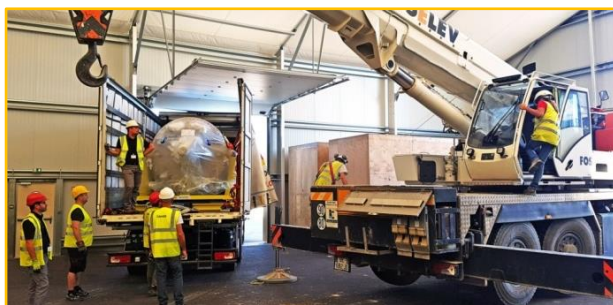
FIG. 5: The pre-production cryopump was delivered in August 2017. More than 15 companies in Europe were involved in its manufacturing.
