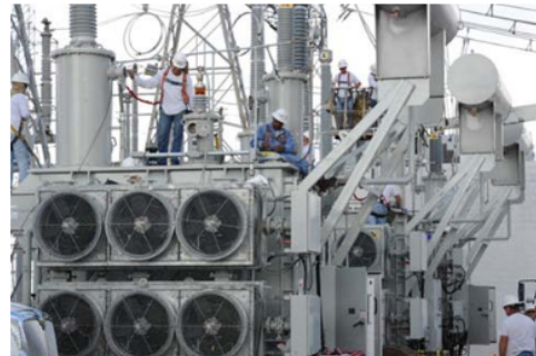
RecX in-grid deployment (Paul Wedig)
