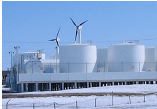
Two of three wind turbines can be seen over the bulk fuel tanks of the Kasigluk Power Station, a vision of what could be possible in the future.
