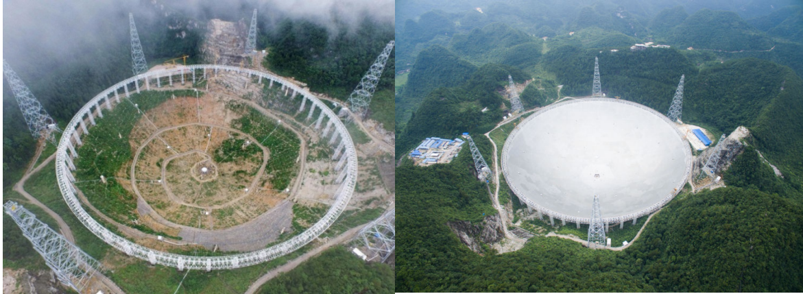
Figure 2: (LEFT) Five-hundred-meter Aperture Spherical Telescope (FAST) under construction in Guizhou Province in 2011. (RIGHT) Completed FAST telescope photographed in July 2016 with all panels installed. FAST operation is scheduled for September 2016, with one of the scientific goals to conduct a sensitive SETI program. (Photo Credit: News.cn).
